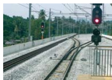
Signalling work, Malaysia - IRCON project.
