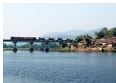
Ro-Ro train crossing the Savitri river bridge at Dasgaon near Veer Station on Konkan Railway route.
