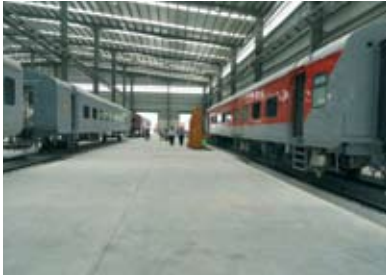
Rail Coach Factory, Lalganj, Rae Bareilly - IRCON project.
