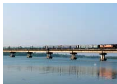
Train crossing the Sharavati river bridge at Honnavar on Konkan Railway.
