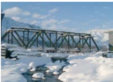
Ready for launch – bridge in Jammu & Kashmir - IRCON project.
