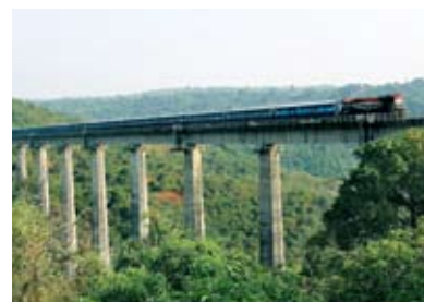
Train crossing the Panvel viaduct on Konkan Railway route.
