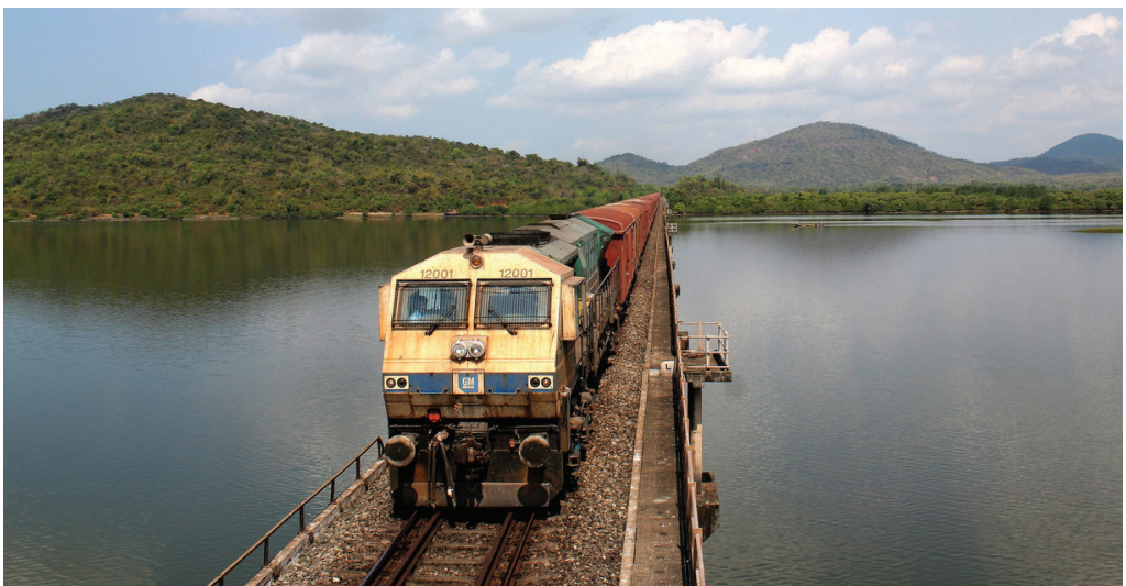
Goods Train Crossing Kali Bridge near Karwar Station at Karnataka KRCL
