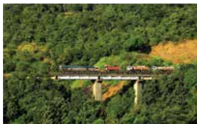
Ro-Ro Train crossing bridge between Ukshi & Sangmaeshwar Station, KRCL
