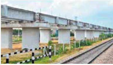
Construction of Viaduct at Renwal in Western, DFCCIL
