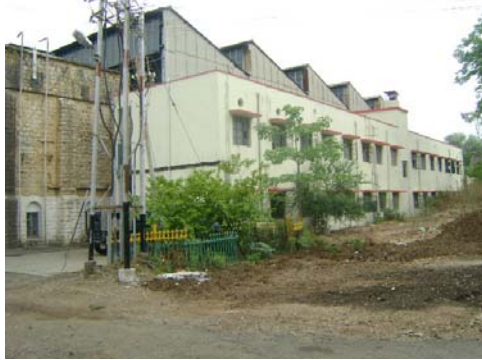
Photo of Shed
