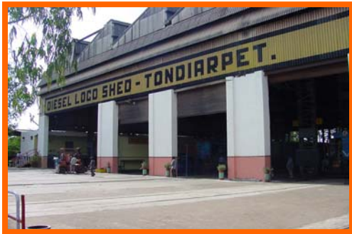
Photo of Shed
