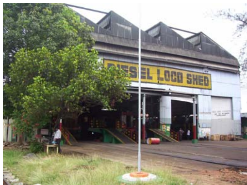
Photo of Shed
